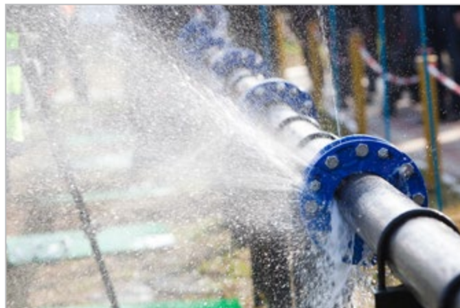
This metal piping system was assembled using a PTFE gasket which exhibited stress relaxation over time resulting in leak paths.
