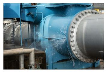
Pipe flange with a polymer seal that failed due to stress relaxation.
