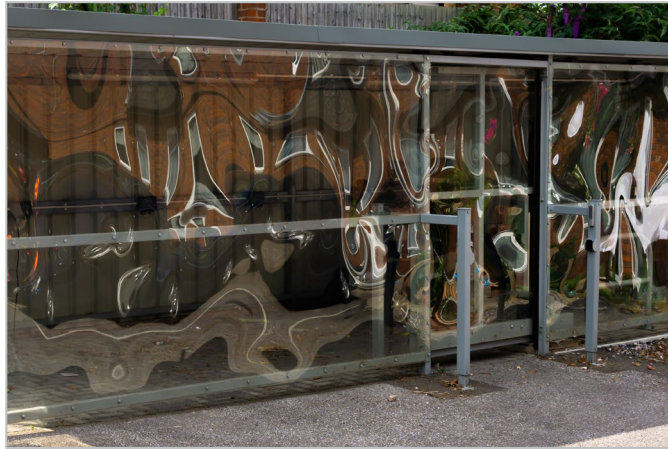
CTE mismatch between the steel structure and the acrylic glazing caused the plastic to warp in warm summer conditions.
