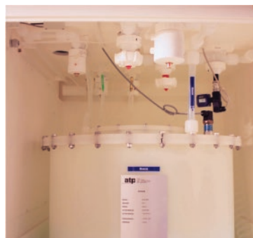
SIMONA® PVDF and SIMONA® PP-H AlphaPlus®: Chemical supply system
